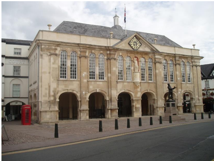
Figure 29 - Shire Hall, Monmouth
